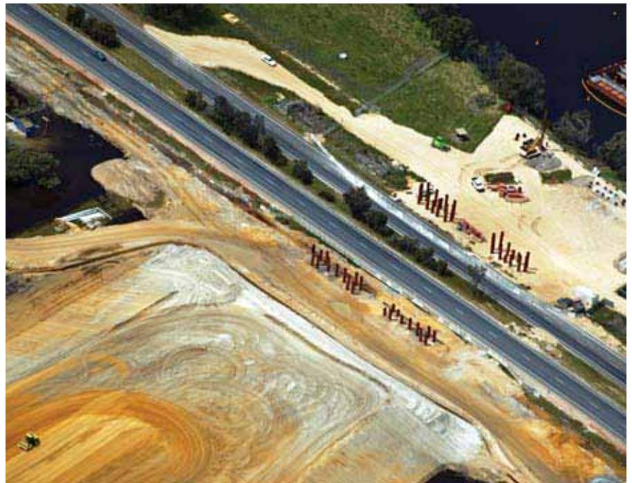
Above – Construction of the Murray River bridge.
