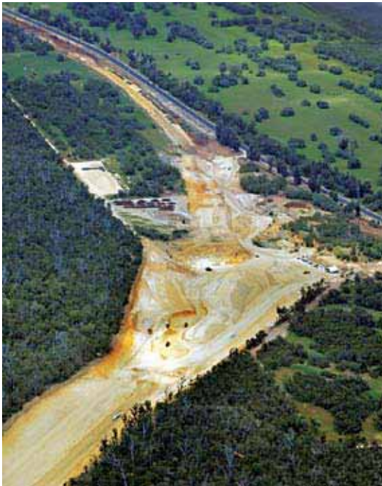
Above – The end of the project, Old Coast Road, looking south.
