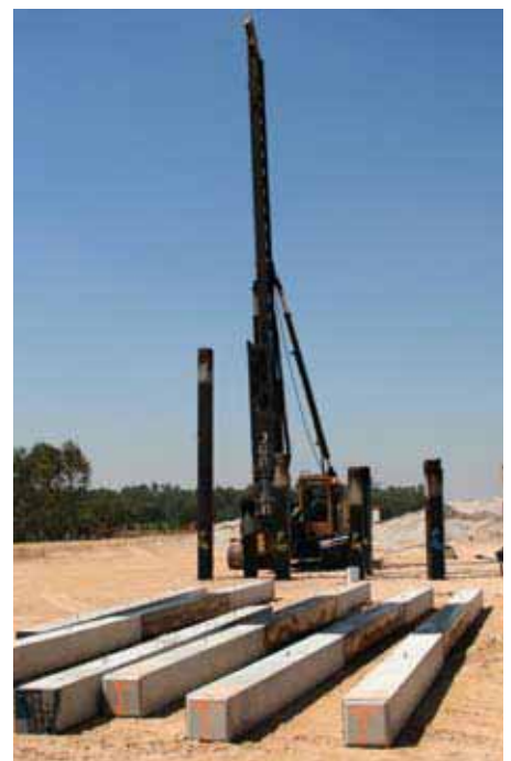
Below – Piling at South Yunderup Bridge
