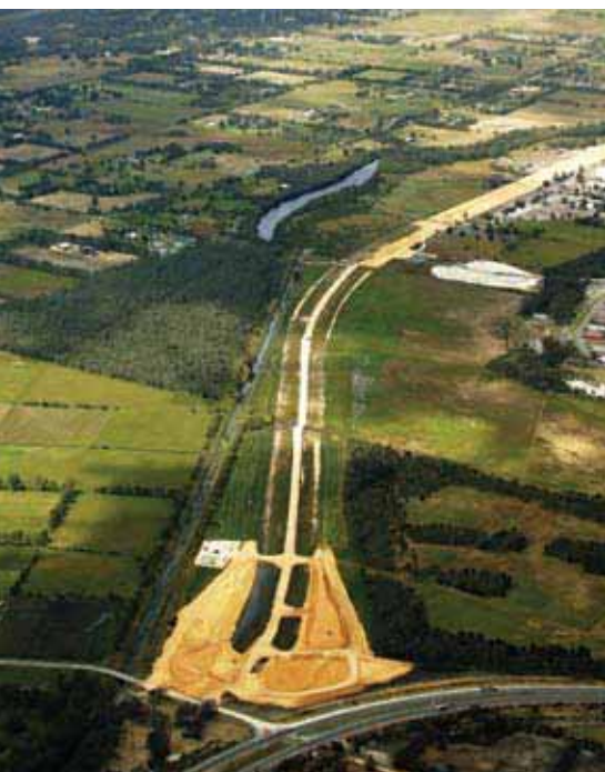
Above – The start of the project, Safety Bay Road interchange, looking south.
