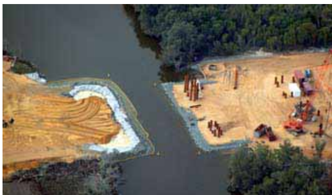
Construction of the Serpentine River bridge
