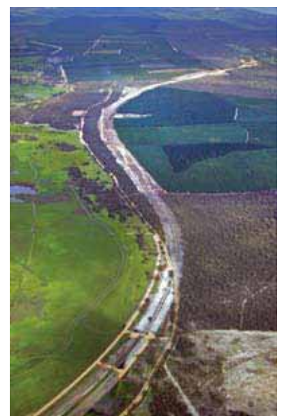
An aerial view of southern section of the NPBH
